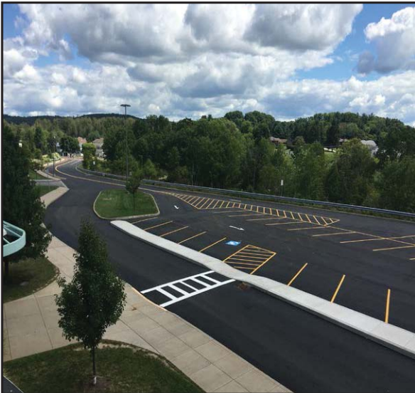
Parking lots and bus loop are complete at George F. Johnson.
