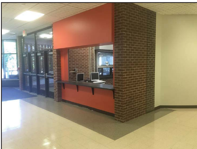
The new High School secure vestibule and information office is complete.
