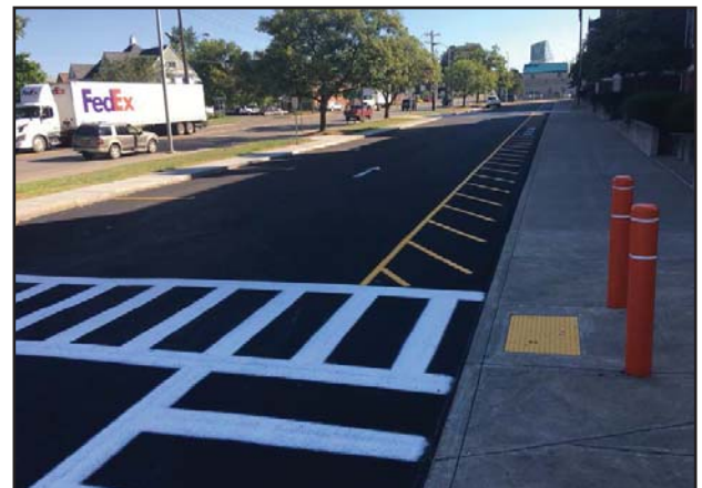
The High School bus loop has been reconstructed.
