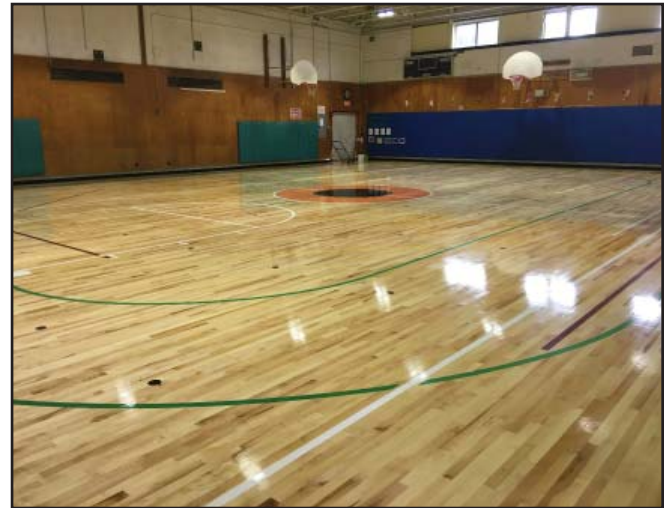
The Charles F. Johnson gym floor has been replaced and a new folding partition installed.
