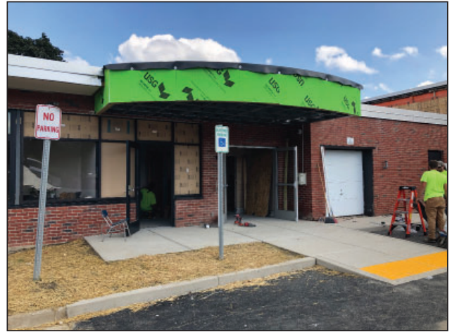
Main entrance at LWW being constructed.
