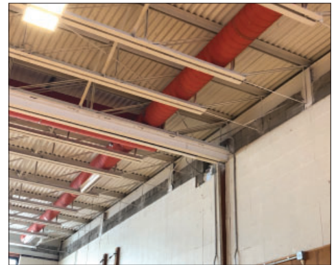
New ductwork installed at LWW gym.
