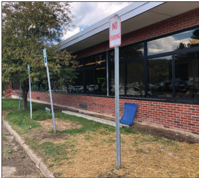
New windows installed at LWW.
