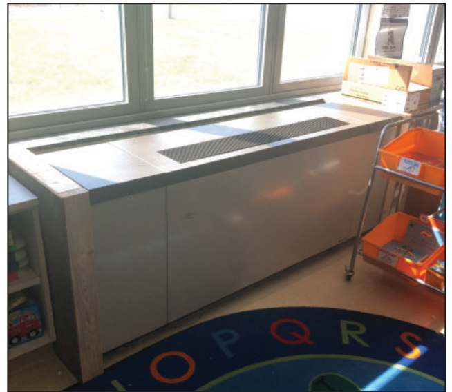
New unit ventilators at CFJ classrooms.
