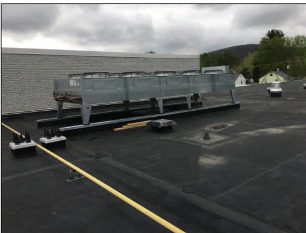
A new condensing unit has been installed on the roof of Charles F. Johnson.
