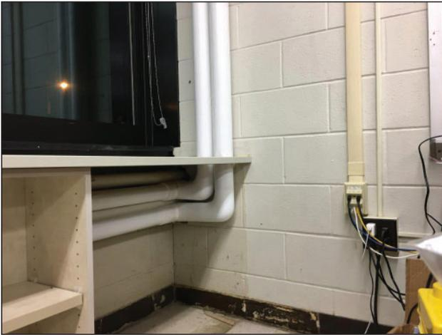
Chilled water piping for air conditioning has been installed at Thomas J. Watson.
