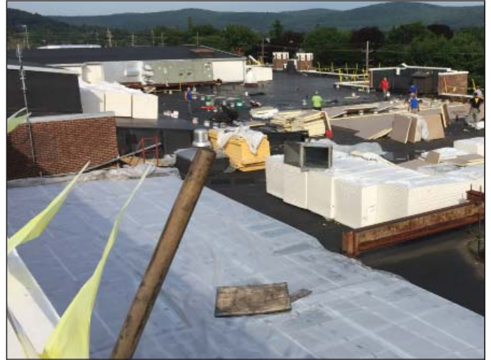
Roof replacement at the High School is progressing.
