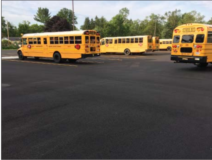
Pavement work at the Bus Garage is complete.
