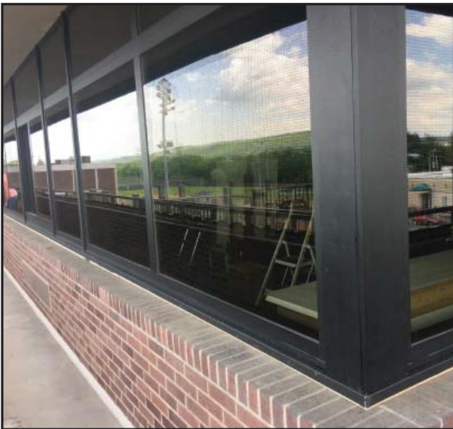
High School windows will continue to be replaced over the summer.
