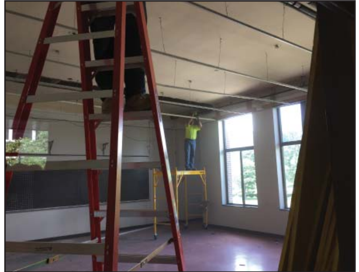
Ceiling replacement has begun at the High School.
