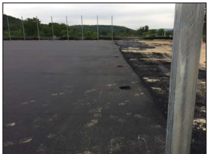
The new tennis courts at AGM are nearly complete.
