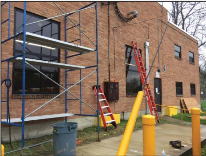
New windows at the Bus Garage have been installed.
