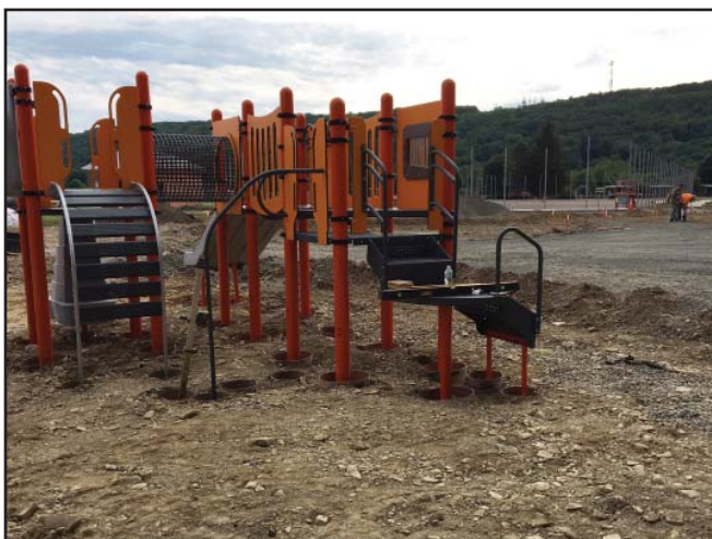
The new playground at AGM is being installed.
